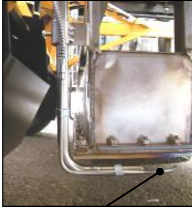
35 - Pilot Thermocouple (one strapped to each pilot)
