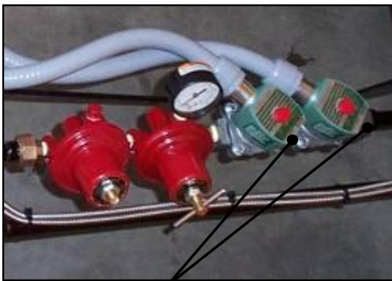
45 - Solenoid Valves (“normally closed” – i.e. electrical power is needed to open them)
