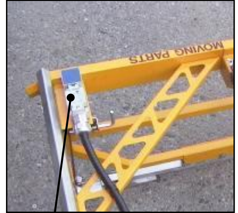
33/34 - Proximity Switch (only forward one shown)
